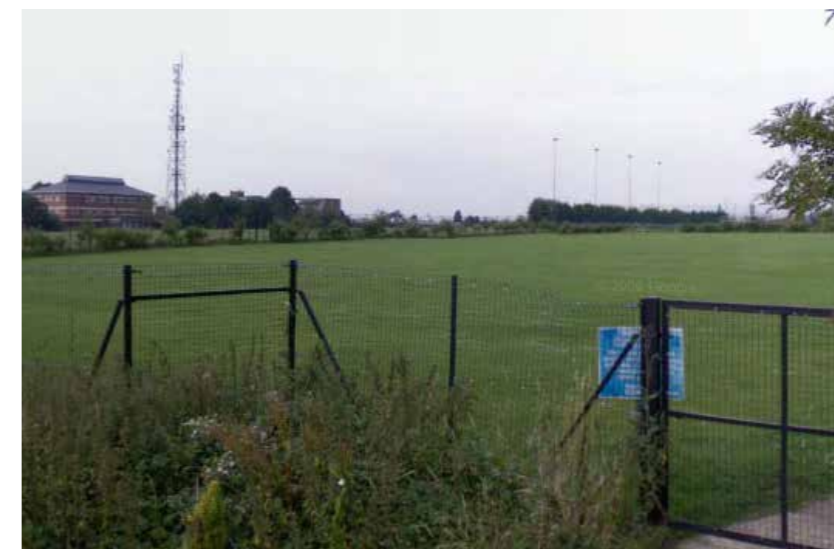
Figure 2.21 Gosford- recreation ground
