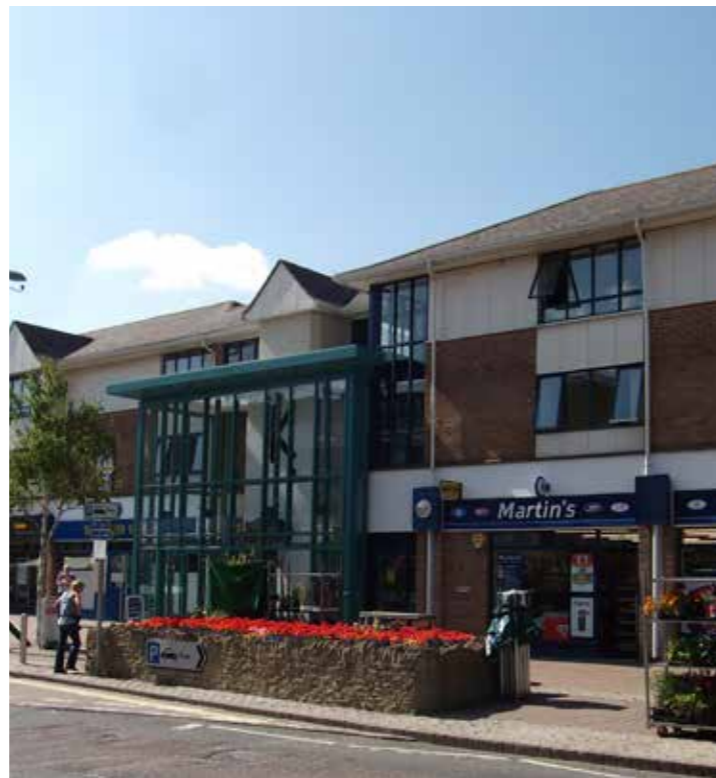
Figure 4.13 Entrance to the
