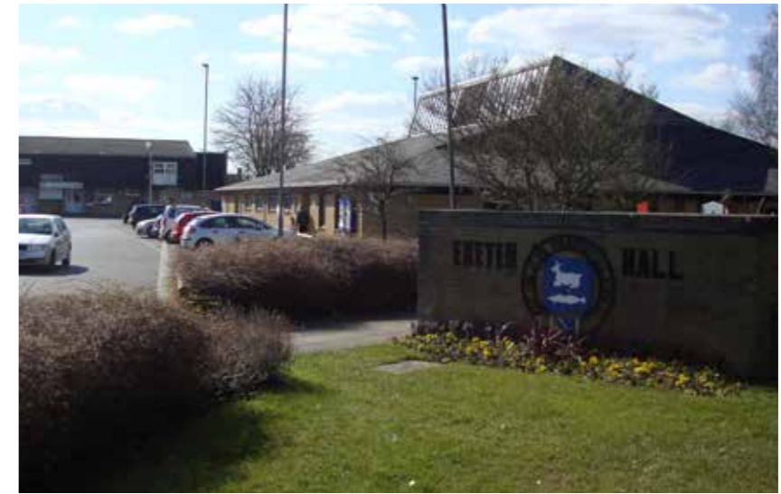
Figure 2.12 Village centre- Exeter Close
