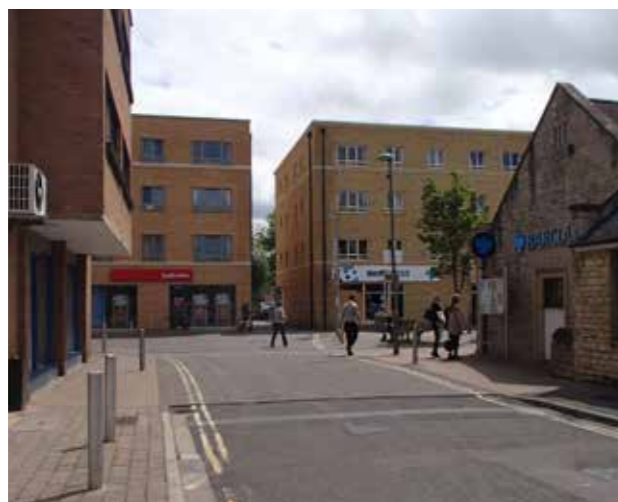
Figure 4.17 Poor quality design of prominent recent schemes
