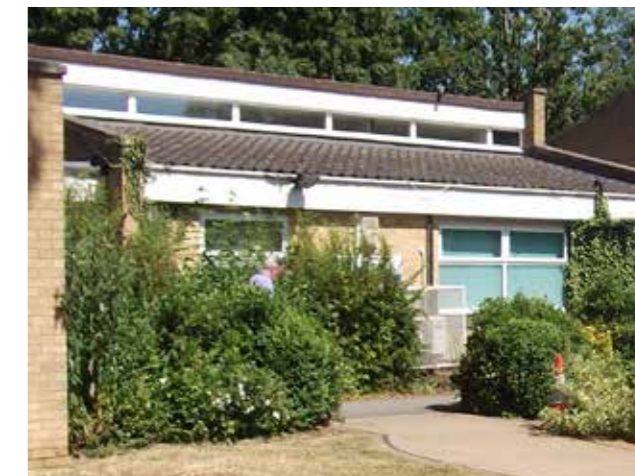
Figure 4.7 Health centre, Exeter Close
